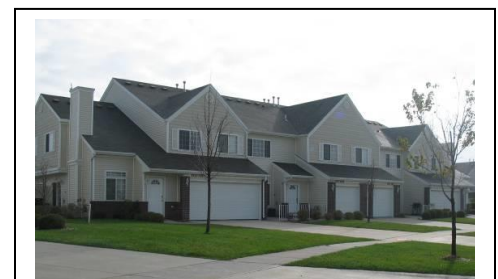
Example of Single-Family Attached
